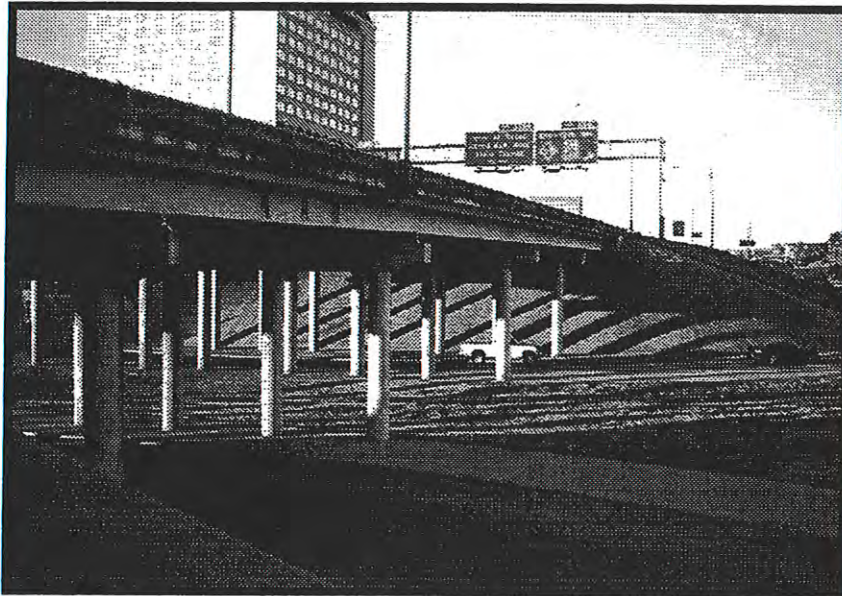
Figure 7: Interstate 35 Separating the Neighborhood from Downtown
